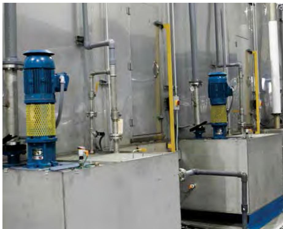
Pneu-Mech manufactures custom washers for surface preparation. As a component in a finishing line, Pneu-Mech washers remove oil, grease and other contaminants from the manufacturing process prior to the application of a wet or powder finish.
